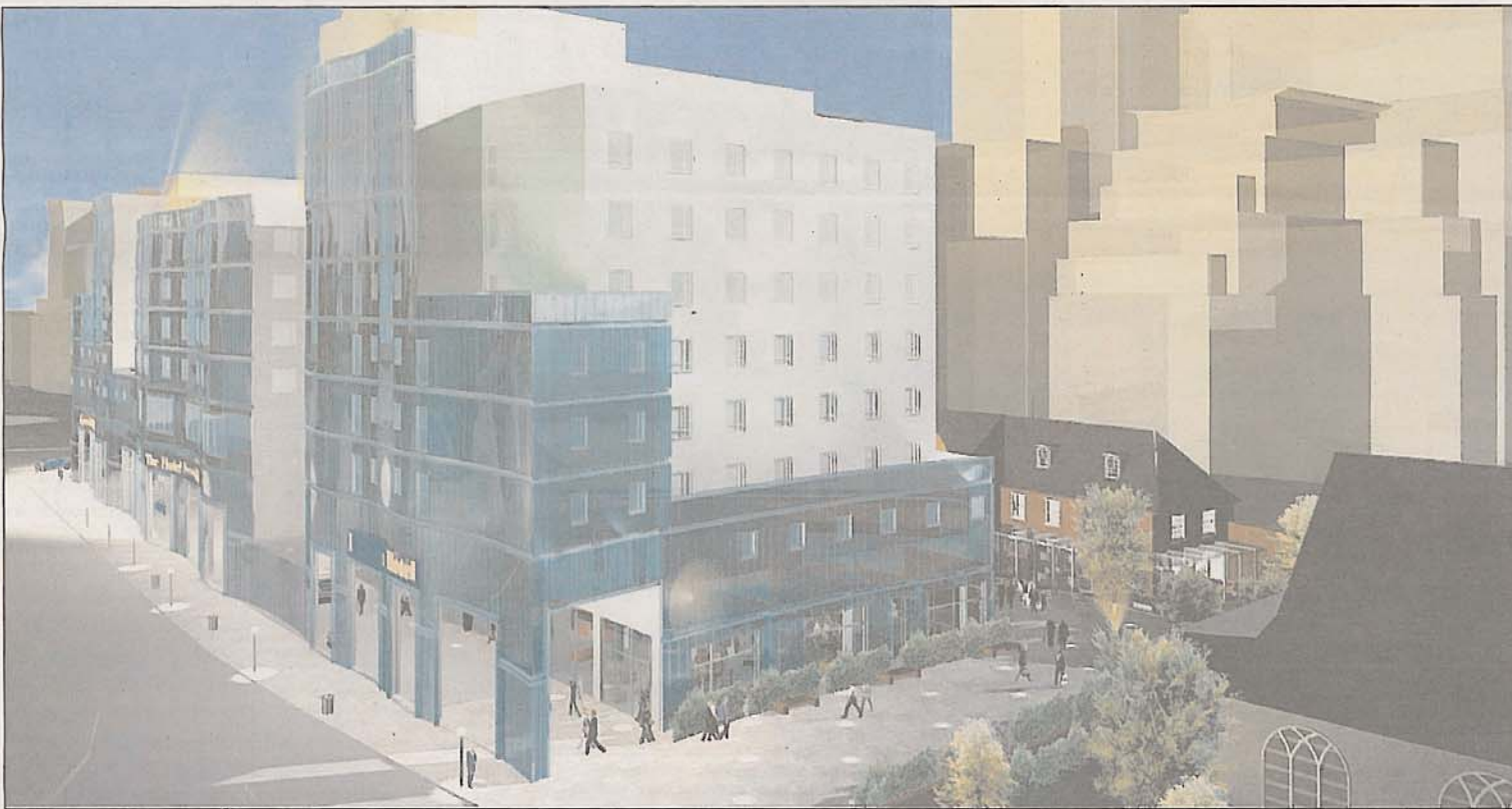
GREEN GLASS: The Star Lane frontage of the proposed St Peter's Port development in Ipswich, with the Waterfront regeneration area in the background
